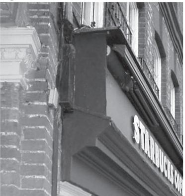
fig 46 canopy beneath cornice & shutter behind fascia
